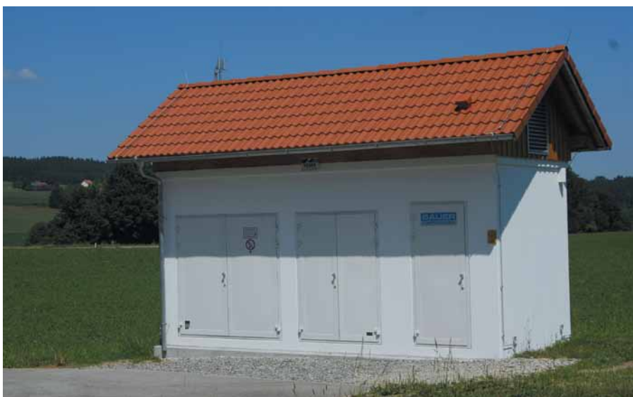
The BAUER compressor station fits perfectly in the Allgäu landscape.
